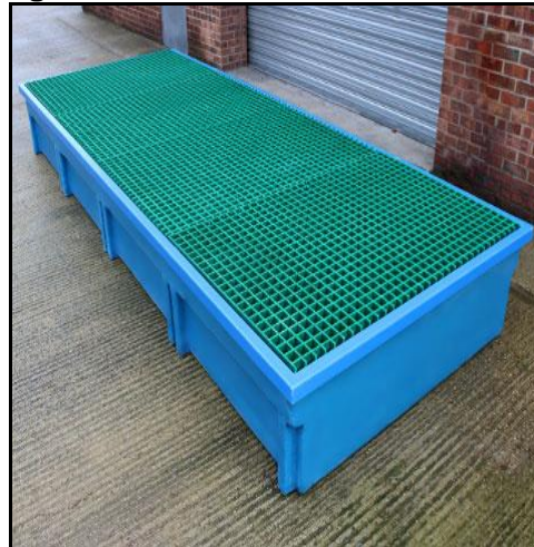
Figure 3 Bund for waste oil container storage
